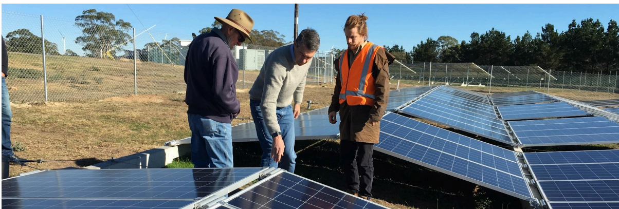
We investigated multiple panel systems before choosing a fixed north with a battery. Here we examine the 5B trial project outside Bungendore with Chris McGrath 5B CEO in early 2018.
